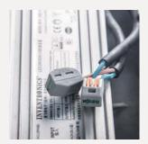
Use German WAGG connectors for internal wiring, safe, convenient & fast.
